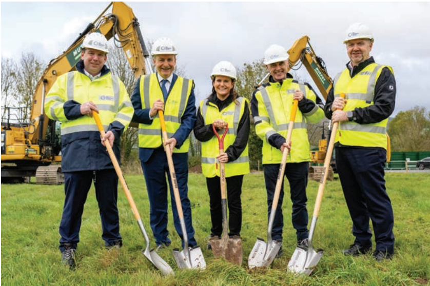
Photographed in October 2024, then-Tánaiste Micheál Martin TD turns the sod to launch construction of Gas Networks Ireland's €32 million Mitchelstown Biomethane Central Grid Injection facility, pictured with David Kelly and Gas Networks Ireland colleagues Brian Sheehan, Edwina Nyhan, and Cathal Marley.
