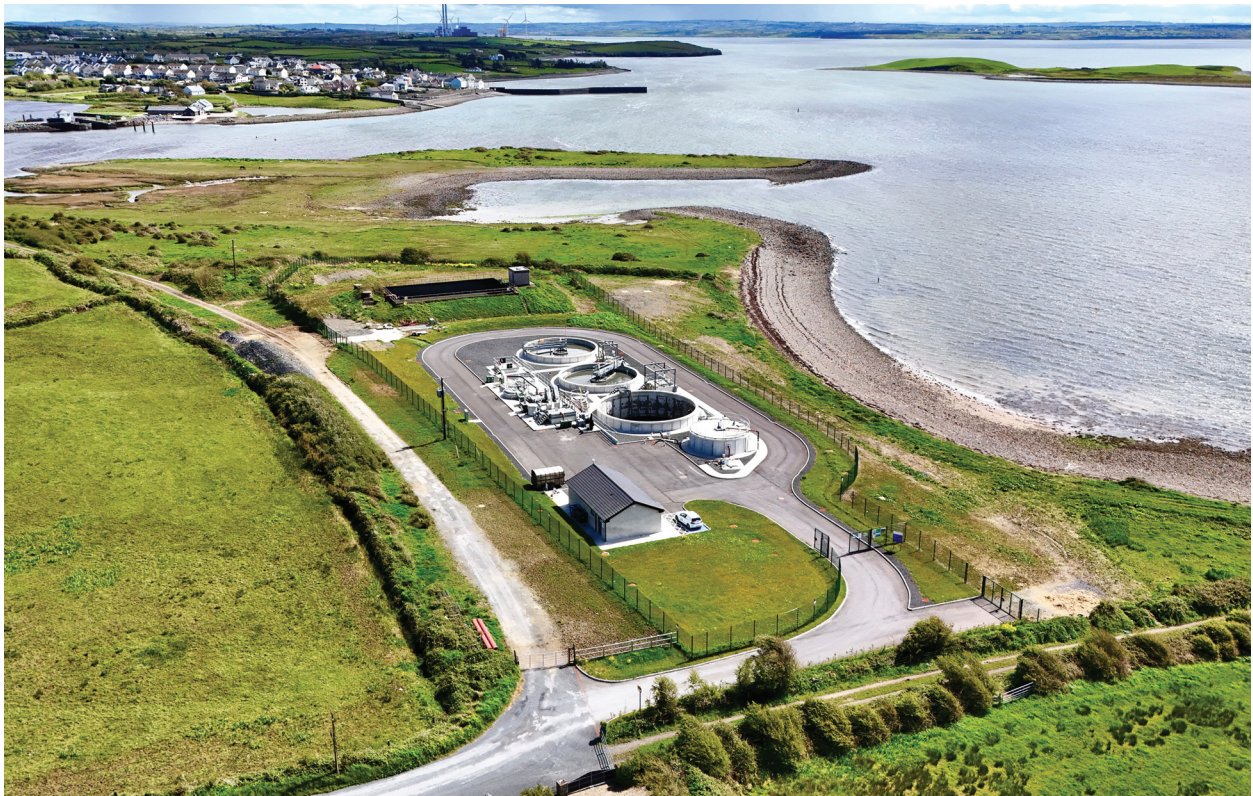
The Kílursh wastewater treatment plant on the Lower Shannon Estuary which was completed in 2024 following an investment of €11 million by Uisce Éireann. Kílursh is one of 35 locations where projects have been completed to date by Uisce Éireann to end the discharge of raw sewage.
