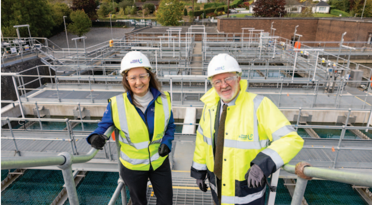
Maria O'Dwyer pictured with the then-Minister of State Malcolm Noonan at the official opening of the new Troyswood Water Treatment Plant in Kilkenny in October 2024.
