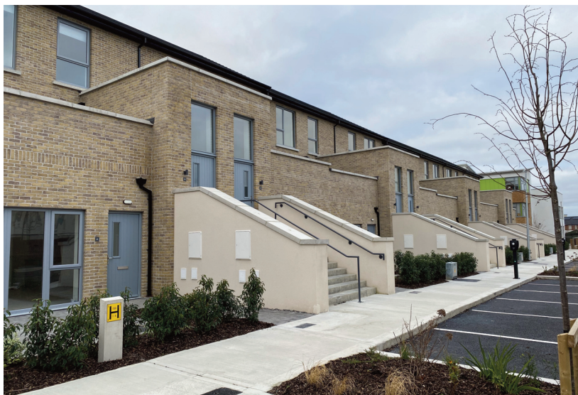
Residents will shortly be moving into the mixed tenure development at Parkside, Belmayne, County Dublin.
