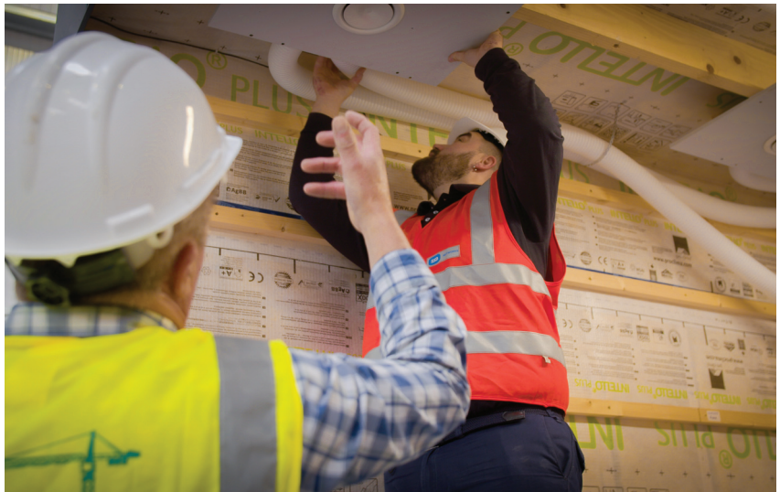
Electrical Apprentice, Adrian Bolger, at Mount Lucas.
