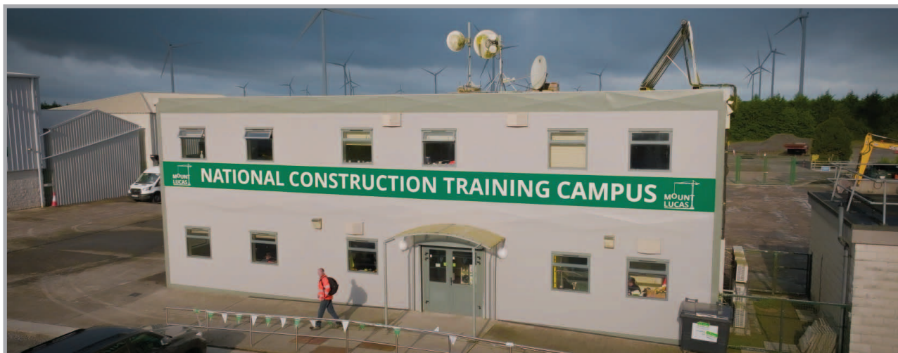
The National Construction Training Campus, Mount Lucas
