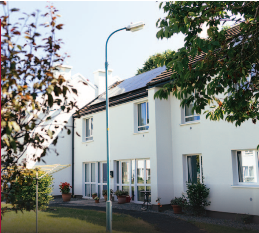
Dún Laoghaire-Rathdown, 2022 retrofit of Beaufort Housing Complex, under the EERP program.
